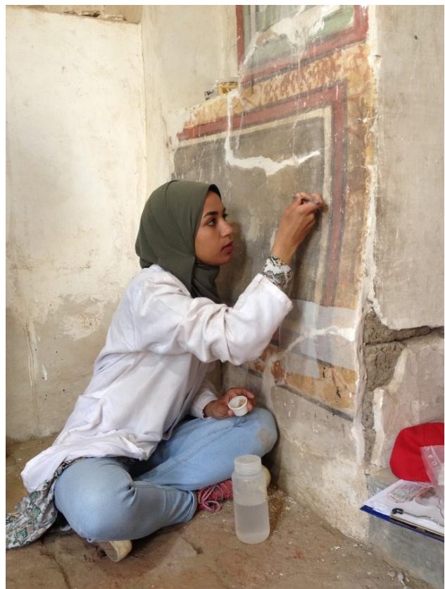
Fig. 8: Field School 2018- Filling cracks at GB 13
