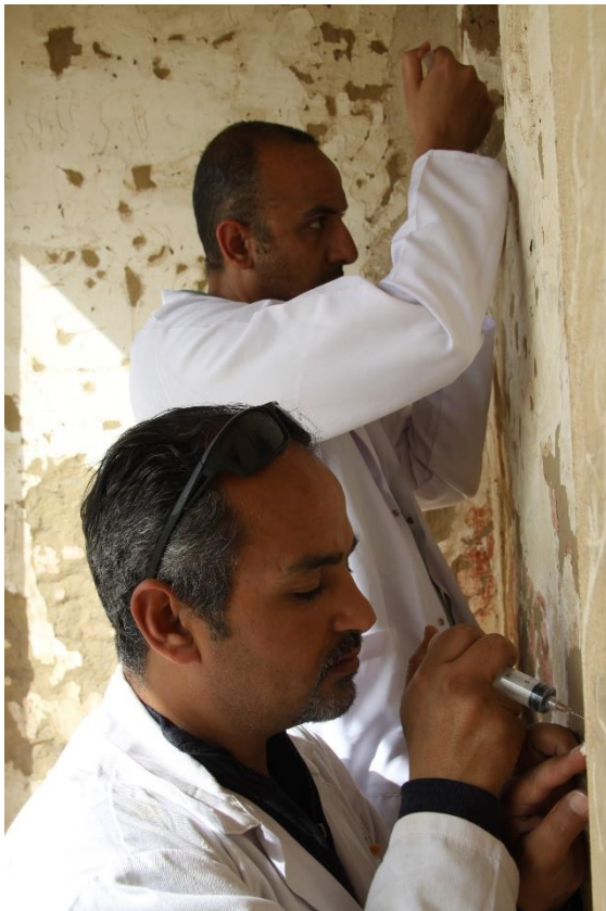
Fig. 7: Field School 2018- consolidation of mud plaster at GB 24
