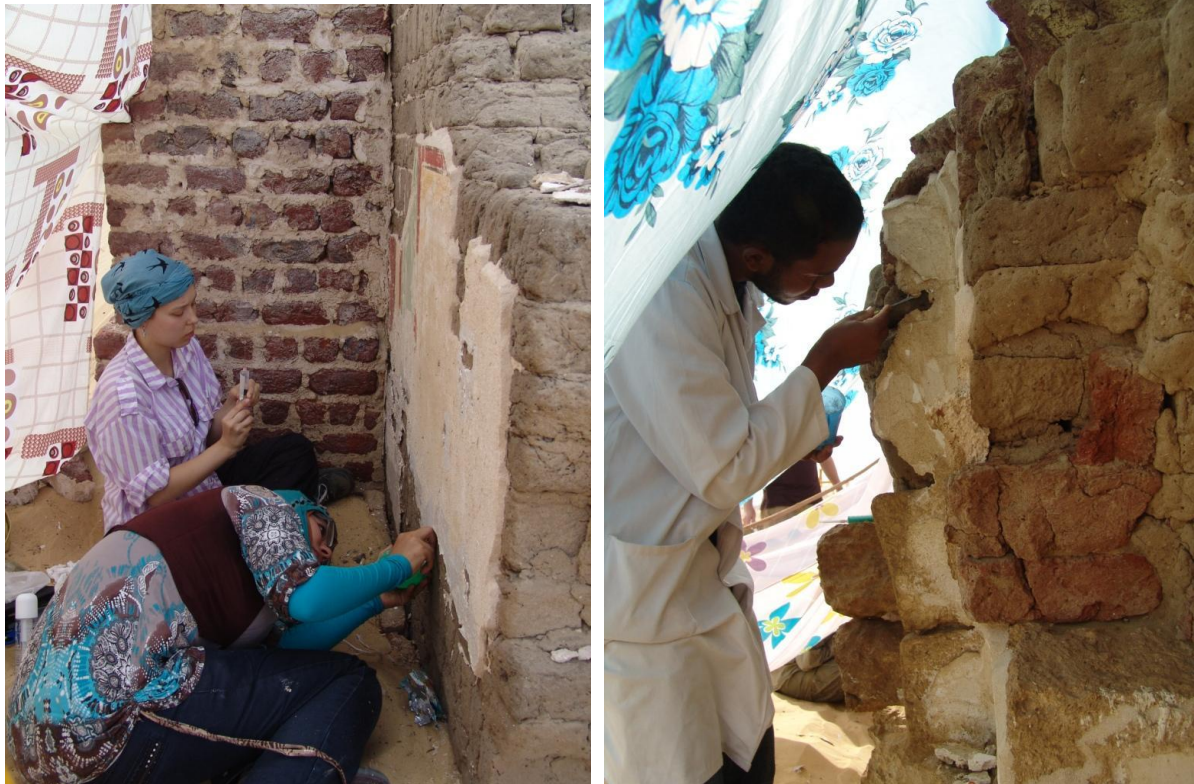
Figs. 5+6: Field school 2012- Plaster conservation at GB 13 (left) and GB 21
